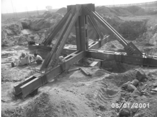
Fig. 2 Footing Load test in Progress
